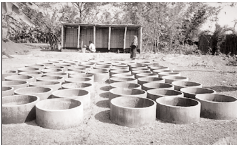
Village Sanitation Center
