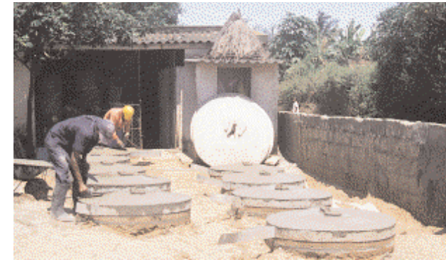
Serial production of dome-shaped SanPlats at the Maxaquene training centre in Maputo. Note that the SanPlats can be cast one on top of the other, hence reducing the need of space at the casting yard.
