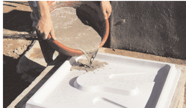
The small SanPlat 60x60 cm is easily made in an all-in-one plastic mould. For best results the first portion of concrete should be a cement slurry. Later much stiffer concrete (1+2+2 volumes of cement, sand and stone) is added to absorb the excess water.
