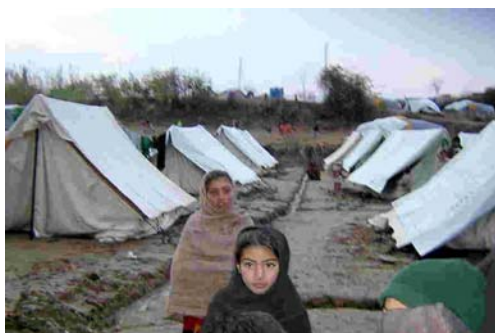
Simple earth drains being constructed to reduce the muddy conditions around the tents in Jabba tented village, IDP camp in Pakistan
