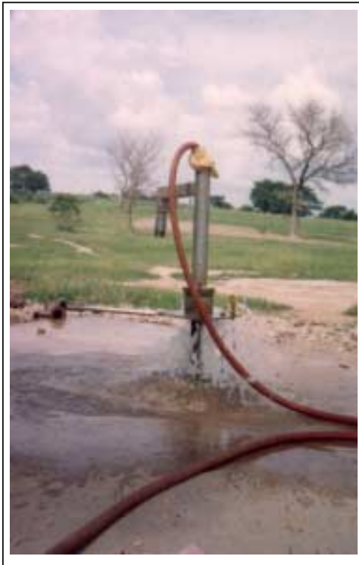
Figure 7: Airlift Blowing & Surging in Progress
