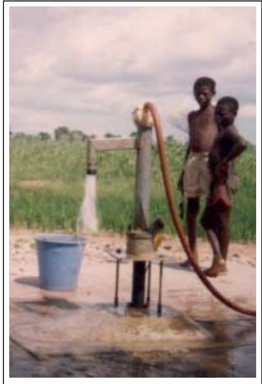
Figure 5: Airlift Pumping in Progress
