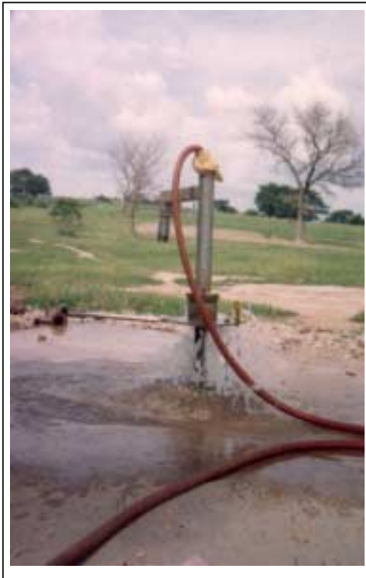
Figure 7: Airlift Blowing & Surging in Progress
