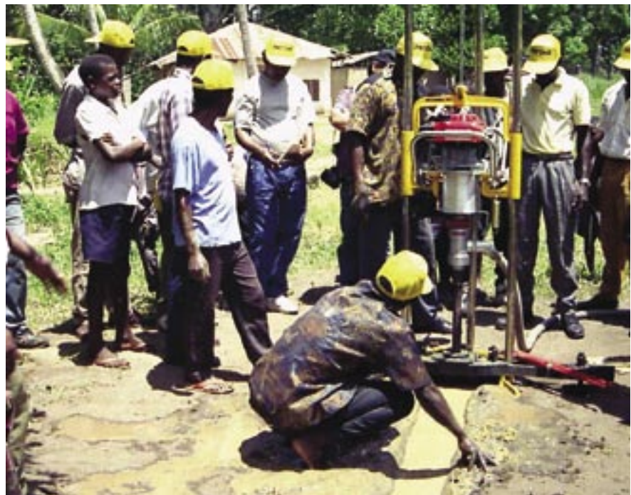
A reduced-diameter drill rig in operation.
