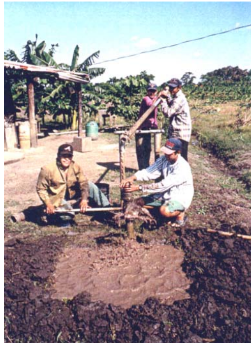
Rota sludge drilling
