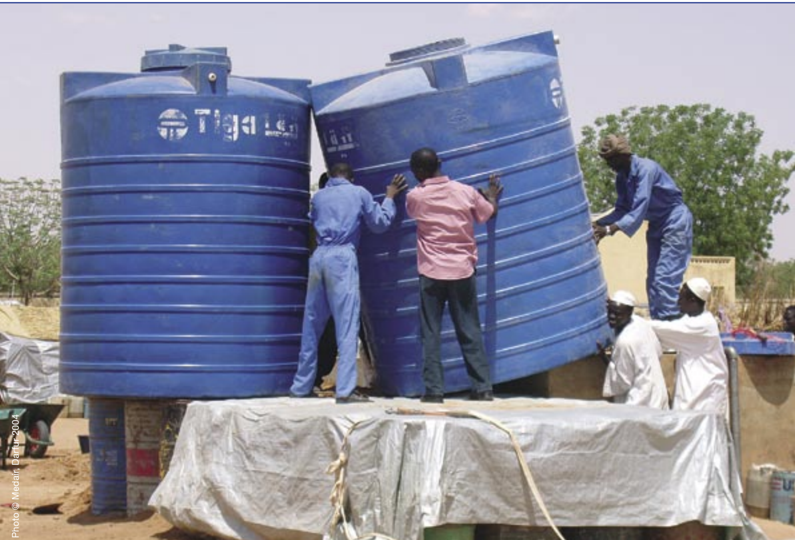
Storage enables sustainable supply
