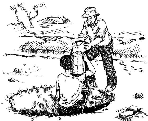
Digging an infiltration well
