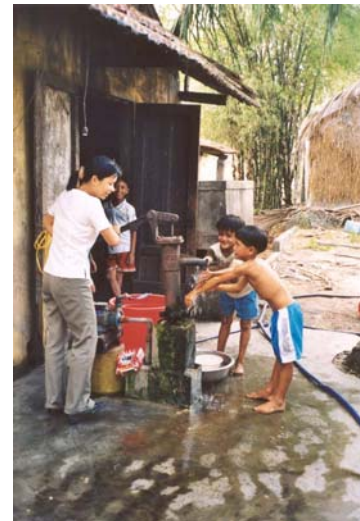
Figure 9 Handpump and Electric Pump on the same borehole
