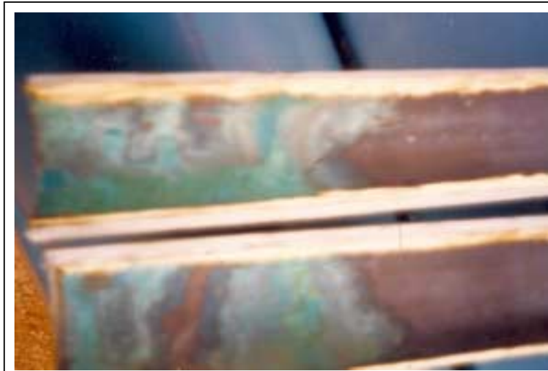
Figure 4. Corroded New Brass Cylinder Linings – Afridev
