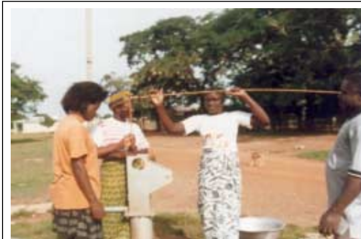
Figure 9. Pump Repairs – Afridev
