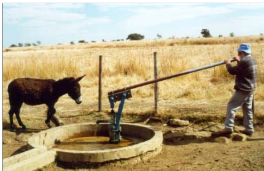
B-Type Bush Pump on borehole
