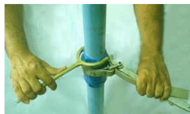
Joining PVC Riser pipes
