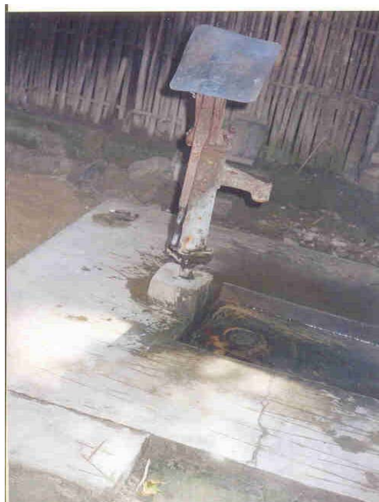
Figure 4.15: Cleanliness of tubewell surroundings improved
