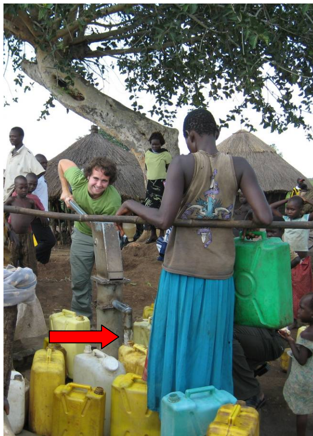
Plate 5 ~ The India Mark 2 delivery tube does not fit Jerry Cans, leading to the use of dirty plastic funnels and poor hygiene practice
