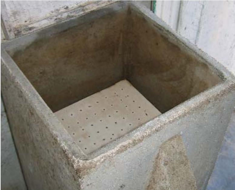
Figure 3.4: A diffuser plate inside a BioSand Filter in the Dominican Republic. Source: Heather Lukacs, 2004.
