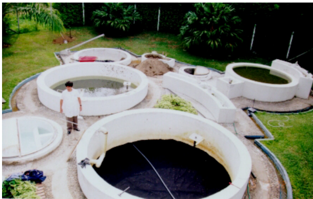
MSF plant with synthetic blankets. Research project by CINARA in Cali, Colombia
