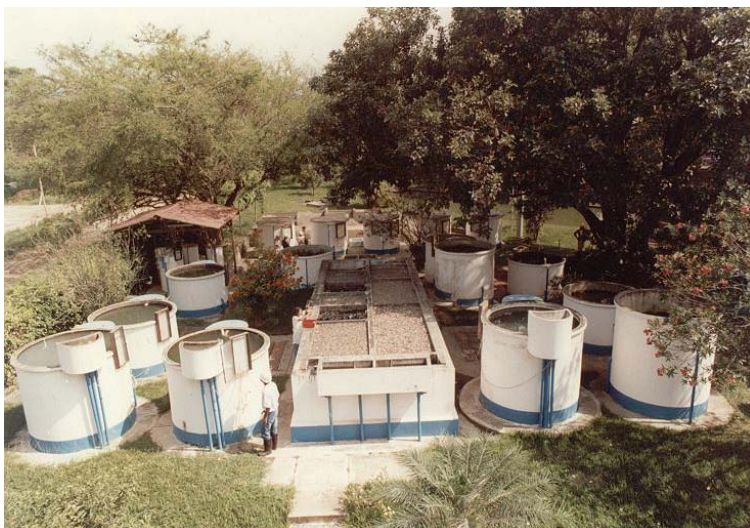
MSF pilot plant units at the Puerto Mallarino research station
