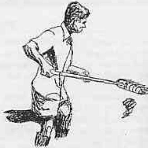
Swab down the filter walls
